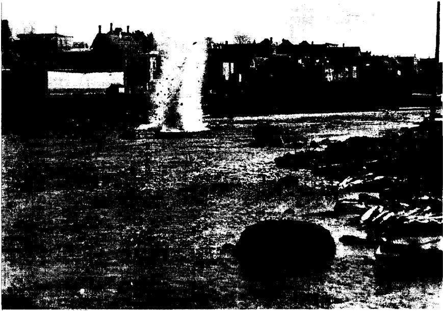
Figure 1. Dredging the Magog River with Dynamite during the Drought of 1903
